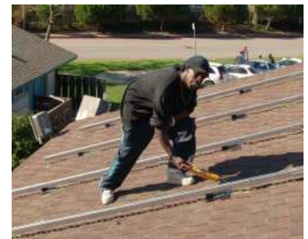
Photos of installation at Golden Gate Village, a Marin Housing property. Left: Front view of installation on Phoenix Project unit. Right: Trainee Garvin Williams installing solar panel brackets on the roof of the Phoenix Project.
