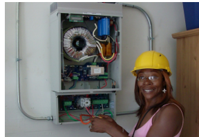
Jacqueline Hall busy working on Wells Fargo Grid Installation.
